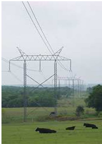
Oncor Electric Delivery
